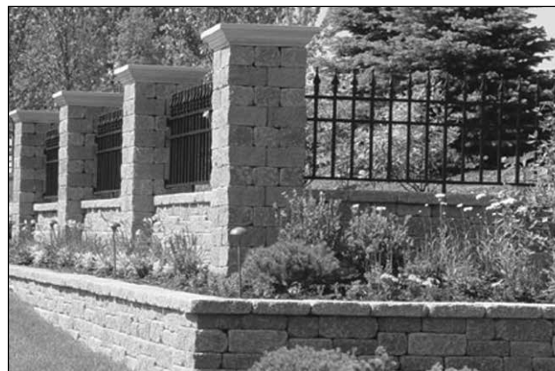
Integral columns within a tiered wall design work well with sections of metal fencing for a creative hardscape design.
