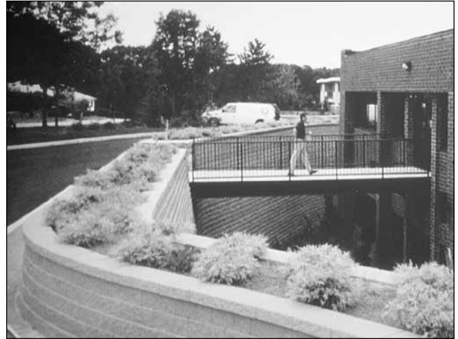
Back-to-back VERSA-LOK walls can act as pedestrian barriers. This design also provided room for planting.
