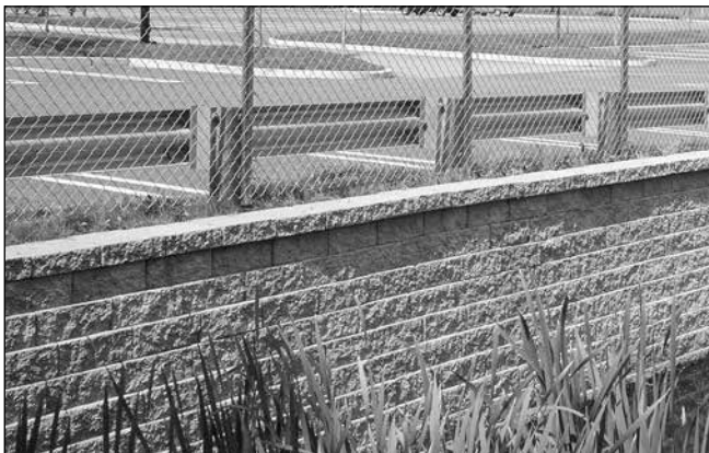
When space allows, fences and railings should be placed several feet behind VERSA-LOK walls.
